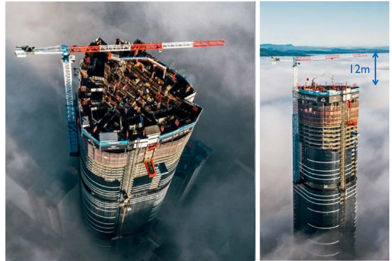
Brisbane Sky Tower 270m building height (pictured under construction) a 12m construction zone beneath the PANSOPS limits or RL335 may be considered reasonable.
